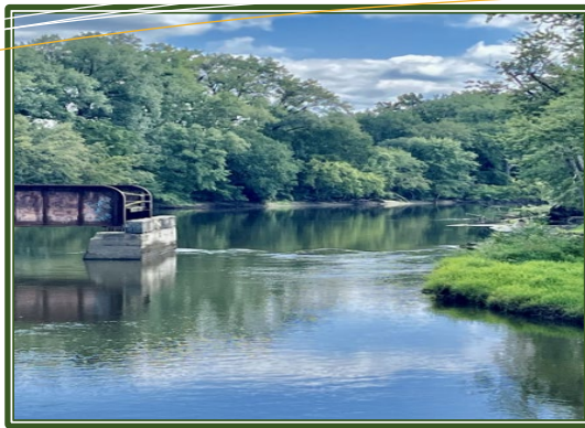
Out-of-service bridge between Lake and Newton Counties following its partial removal (Aug. 2024).
