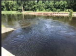
SEAWALL ABSORBS VELOCITY ON OPPOSITE BANK
