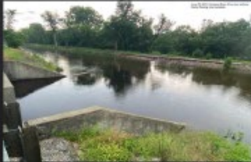
KANKAKEE SPILLWAY (FLOWING OUT), JUNE 29
