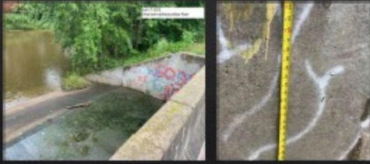
YELLOW RIVER SPILLWAY, JULY 17
