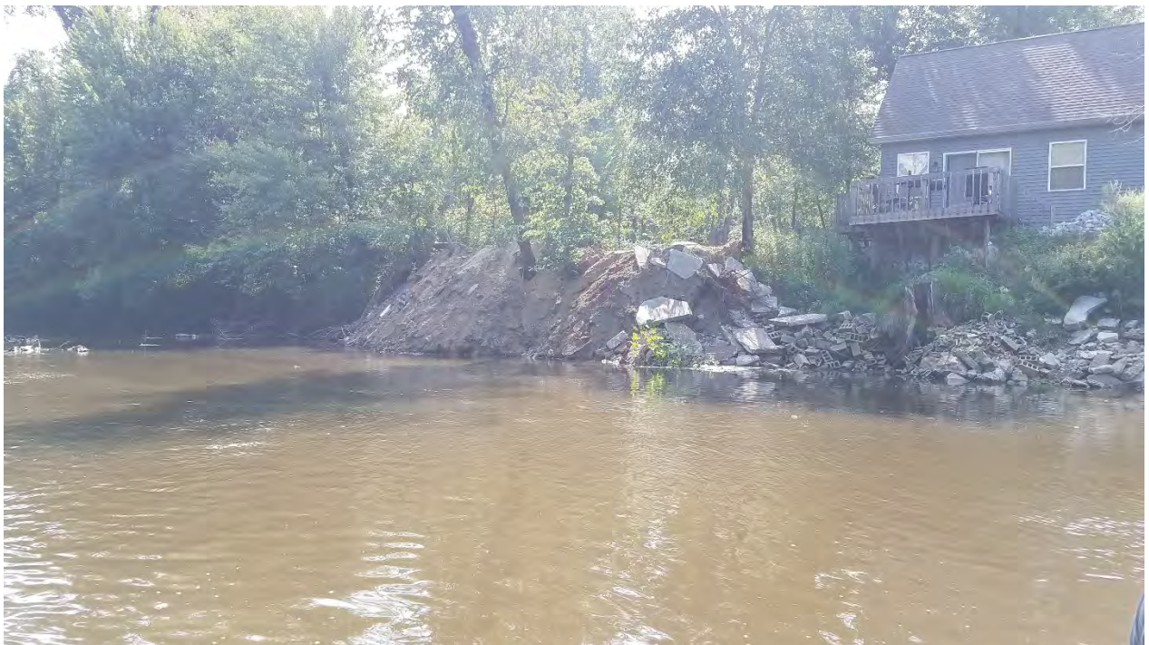
Photo 6: Rubble and Eroding Berm Near Home in Newton County
